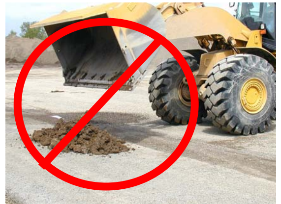
Don't Dump Dirt or Bark Mulch on Pervious Concrete
